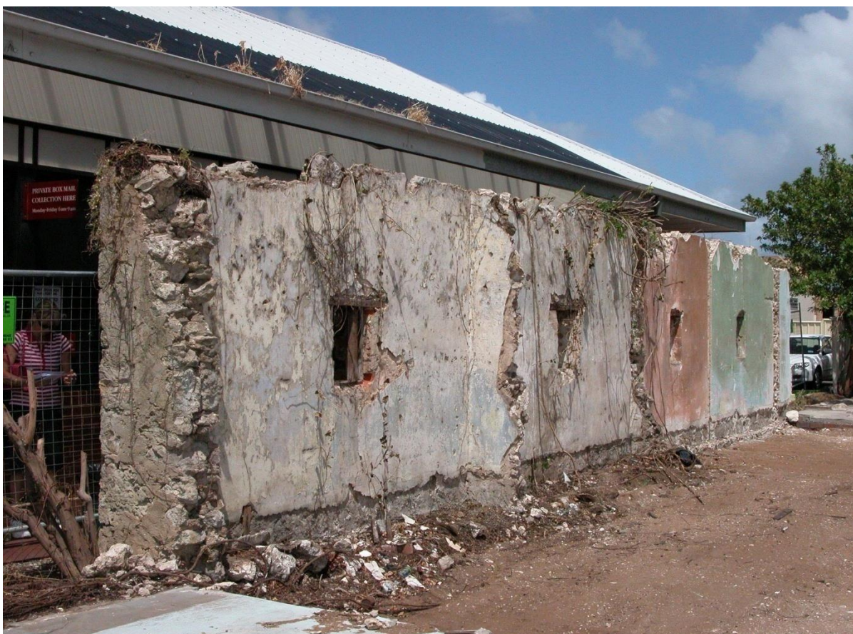
The remaining wall of the Migrant Barracks, next to the post office in Sholl Street. Photograph taken (2011)
