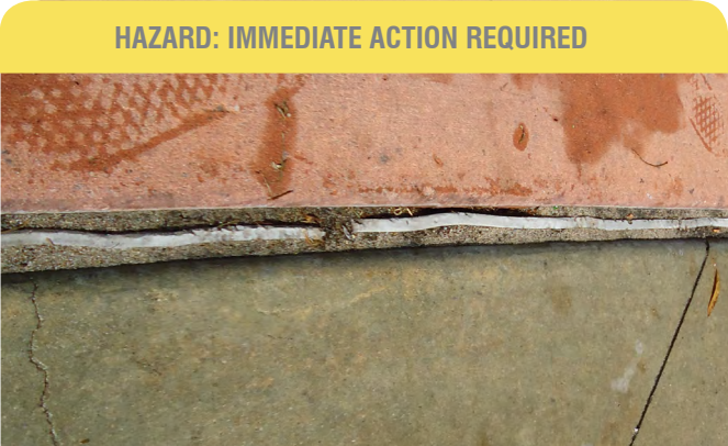
HAZARD: IMMEDIATE ACTION REQUIRED DIFFERENTIAL SETTLEMENT: LARGE GAPS IN BETWEEN ADJACENT CONCRETE SURFACES MAKES IT VERY DANGEROUS FOR SKATE AND SCOOTER USERS TO TRANSITION OVER. IMMEDIATE ACTION IS RECOMMENDED TO RECTIFY THIS ISSUE.
