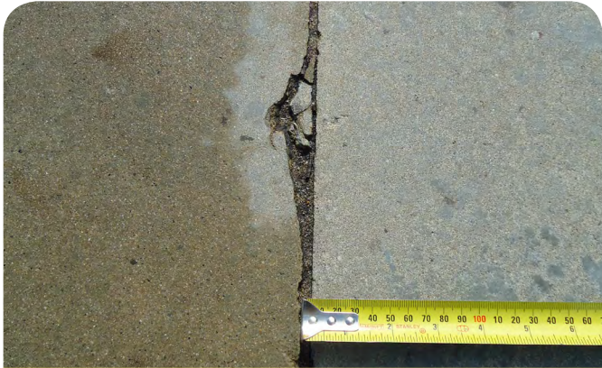
CHIPS AND CRACKS: THERE ARE A FEW LOCATIONS OF MINOR CHIPS AND CRACKS, HOWEVER THESE CURRENTLY DO NOT APPEAR TO EFFECT FUNCTION, STRUCTURAL INTEGRITY OR SAFETY. BUT ALL CHIPS AND CRACKS SHOULD BE CONTINUALLY INSPECTED.
