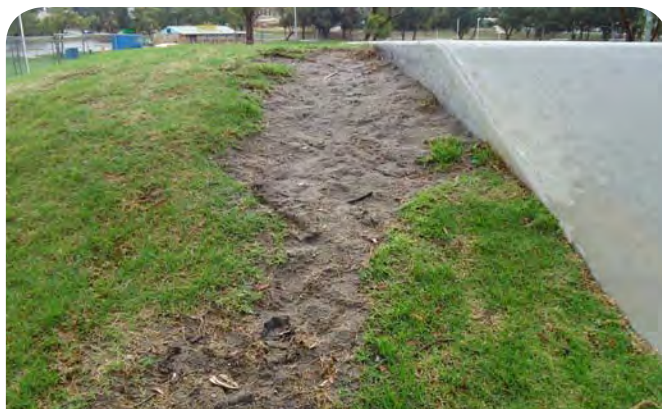
EROSION: THERE ARE LARGE SECTIONS WHERE FOOT TRAFFIC IS CAUSING THE EROSION OF THE EMBANKMENT INCREASING FALL HEIGHTS AND POTENTIALLY UNDERMINING THE CONCRETE. IT REQUIRES REPAIR TO ENSURE NO FURTHER DAMAGE IS CAUSED.
