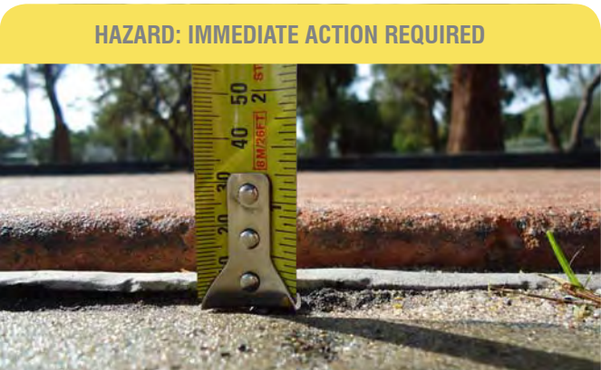
HAZARD: IMMEDIATE ACTION REQUIRED DIFFERENTIAL SETTLEMENT: LARGE GAPS IN BETWEEN ADJACENT CONCRETE SURFACES MAKES IT VERY DANGEROUS FOR SKATE AND SCOOTER USERS TO TRANSITION OVER. IMMEDIATE ACTION IS RECOMMENDED TO RECTIFY THIS ISSUE.
