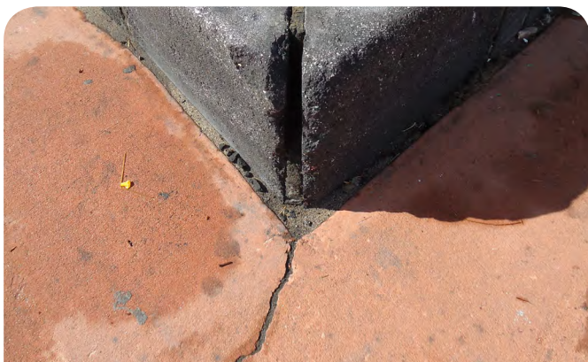
CHIPS AND CRACKS: IT APPEARS THE SEATING TERRACE IS ALSO BEING USED AS A SKATE ELEMENT. IT HAS SUFFERED SOME INCIDENTAL DAMAGE AND IMMEDIATE ACTION IS RECOMMENDED TO RECTIFY THE EXPOSED GAP.
