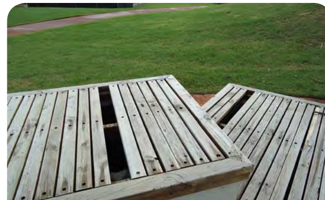
DAMAGE (MALICIOUS): TIMBER SLATS HAVE BEEN PULLED FREE FROM THE SEATING TERRACE. SOME OF THE REMAINING SLATS ARE LOOSE OR SPILT. IMMEDIATE ACTION IS RECOMMENDED TO RECTIFY THE DAMAGE.
