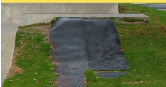
HAZARDS: USERS HAVE ADDED RUBBER MATS TO IMPROVE FUNCTIONALITY, HOWEVER IT IS UNEVEN, SLIPPERY AND THERE ARE LARGE SECTIONS OF SEPARATION BETWEEN THE PLATFORM. IMMEDIATE ACTION IS RECOMMENDED TO RECTIFY THESE ISSUES.
