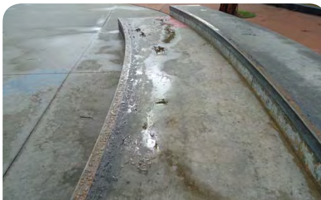
DRAINAGE: SOME LOCALISED POOLING ON THE TWO TIER LEDGE IS PRESENT, HOWEVER THE OVERALL SKATEPARK HAS ADEQUATE DRAINAGE.
