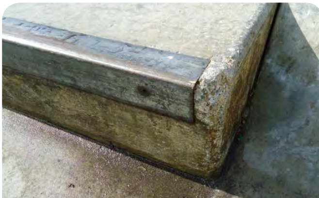
DAMAGE (INCIDENTAL): CHIPPING HAS OCCURRED ALONG THE TOP OF THE MINI RAMP LANDING WHERE THE COPING DOES NOT EXTEND TO THE EDGE. IT REQUIRES REPAIR TO ENSURE NO FURTHER DAMAGE IS CAUSED.
