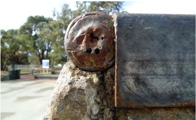
CORROSION: IS APPARENT ON THE CHS COPPING AT THE MINI RAMP ENDS. IT REQUIRES REPAIR TO ENSURE NO FURTHER DAMAGE IS CAUSED.
