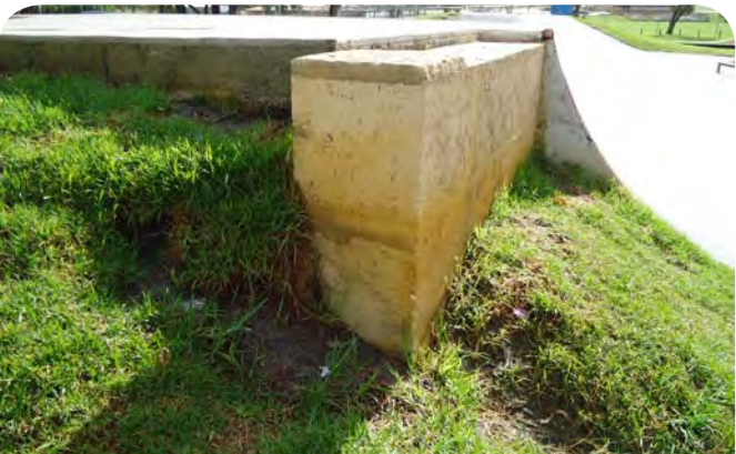
EROSION: THERE ARE LARGE SECTIONS WHERE FOOT TRAFFIC IS CAUSING THE EROSION OF THE EMBANKMENT INCREASING FALL HEIGHTS AND POTENTIALLY UNDERMINING THE CONCRETE & LIMESTONE. IT REQUIRES REPAIR TO ENSURE NO FURTHER DAMAGE IS CAUSED.
