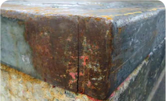
CORROSION: CRACKS ARE APPARENT ON ONE CORNER OF THE TWO TIER LEDGE ALONG THE WELD LINES CAUSED BY CORROSION. IT REQUIRES REPAIR TO ENSURE NO FURTHER DAMAGE IS CAUSED.
