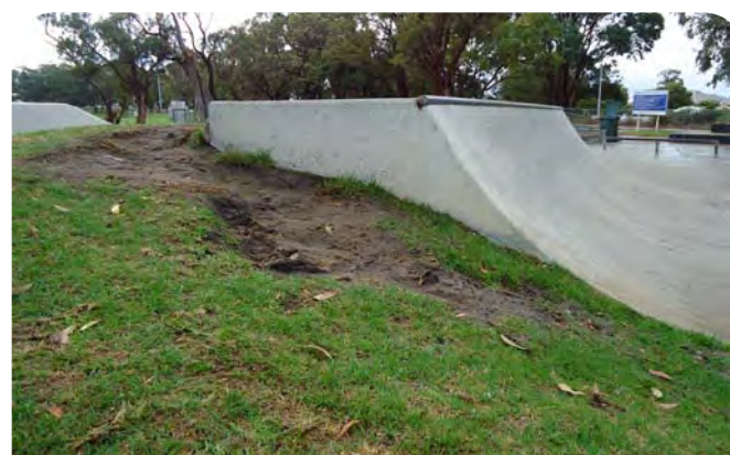
EROSION: THERE ARE LARGE SECTIONS WHERE FOOT TRAFFIC IS CAUSING THE EROSION OF THE EMBANKMENT INCREASING FALL HEIGHTS AND POTENTIALLY UNDERMINING THE CONCRETE. IT REQUIRES REPAIR TO ENSURE NO FURTHER DAMAGE IS CAUSED.
