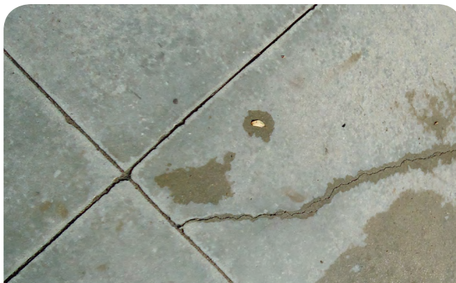
SURFACE FINISH: THE OVERALL SURFACE FINISH OF THE SKATEPARK IS VERY GOOD, DESPITE A FEW MINOR AREAS OF POOLING AND CRACKING.
